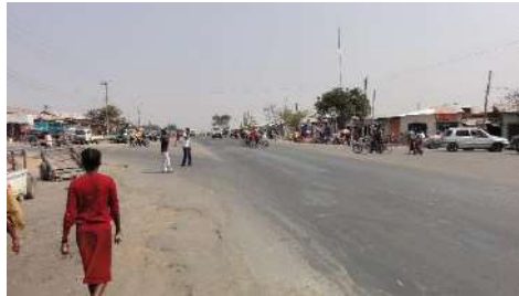
Limited facilities for NMT and no speed calming
