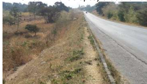
Steep embankment slope
