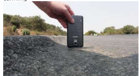
Serious rutting of road
