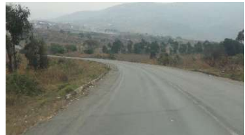
Worn road markings and no delineators or other background markings
