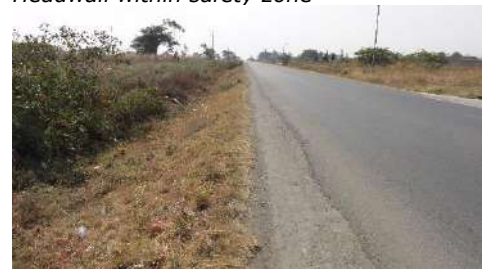
Steep embankment slope
