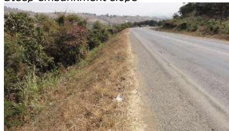
Steep embankment slope
