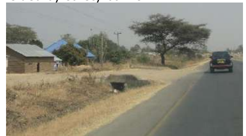
Headwall within safety zone
