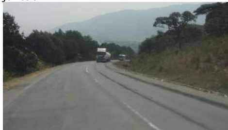
Serious rutting of road
