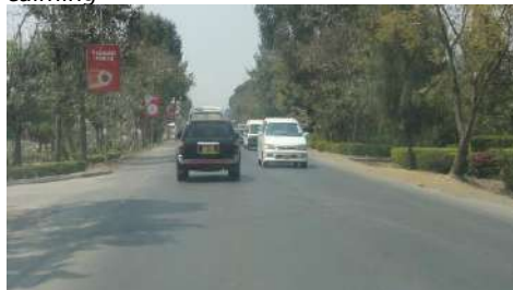
Busy road through town – no marking in junction
